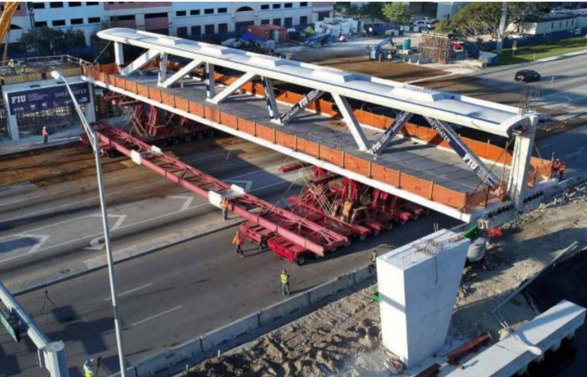
The main span of the FIU-Sweetwater University City Pedestrian Bridge was moved into position over the Tamiami Trail by four motorized lifts on March 10.
