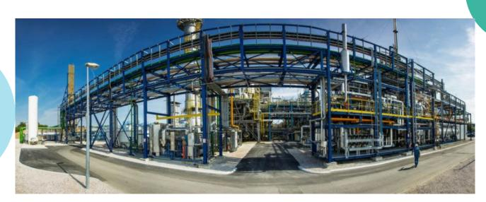
This Cryocap™ unit has an annual capture capacity of 100 000 tonnes of CO<sub>2</sub> at this site.
