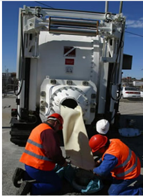
Structural Liner Installation
