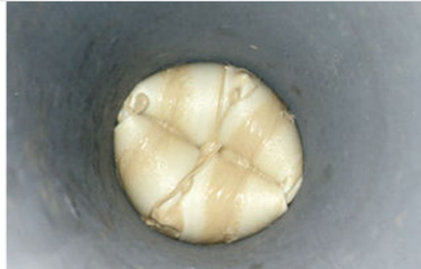
Structural Liner Installation
