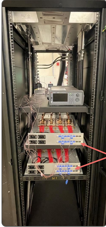
Two-phase in rack CDU system (CDU contributed by VERTIV)
