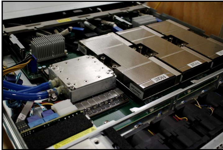
Integration of cooling solution on 1U server
