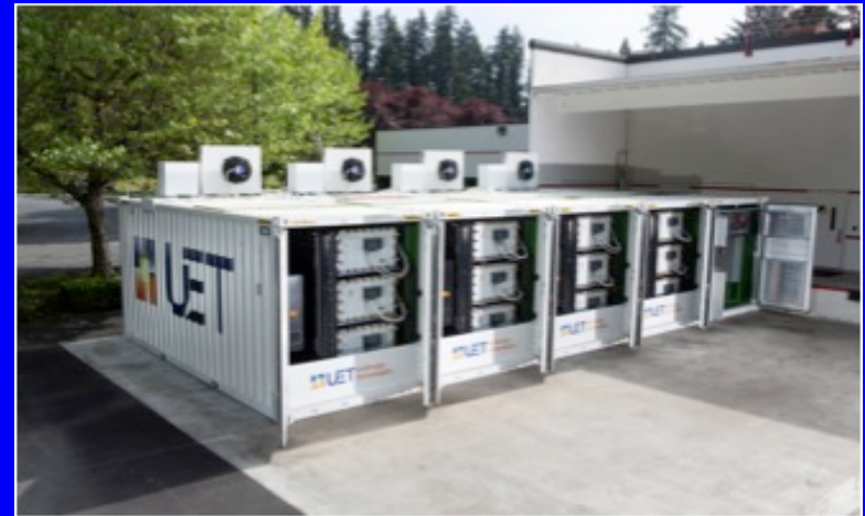
UniEnergy 600 kW/2.2MWh battery system
