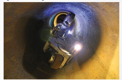
Spray-on polymeric & epoxy systems are being installed robotically. Advanced systems are now able to also apply reinforcement while spraying ->
