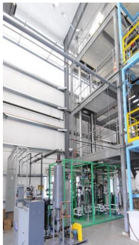
Figure 1: RTI's bench-scale solvent testing unit
